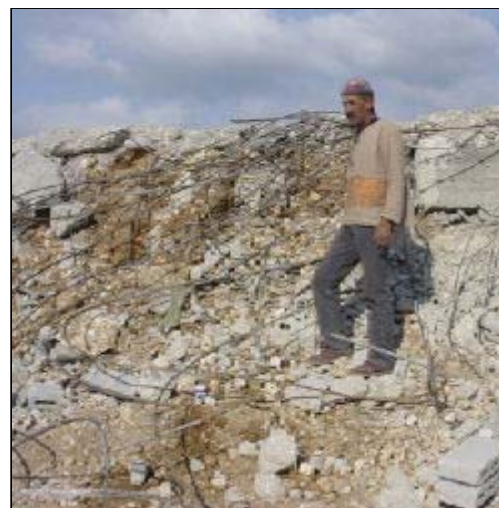
Mohamed Suweid, in front of his demolished house, Im Al-Sahali
